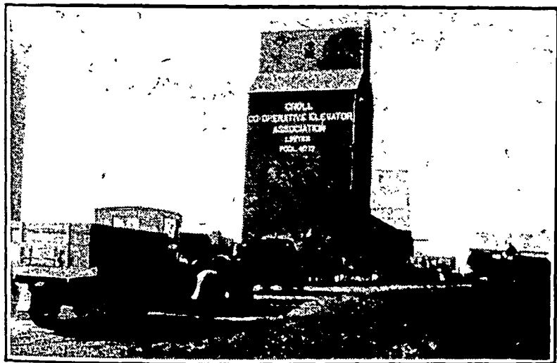
Croll Pool Elevator. A busy spot during the fall season
